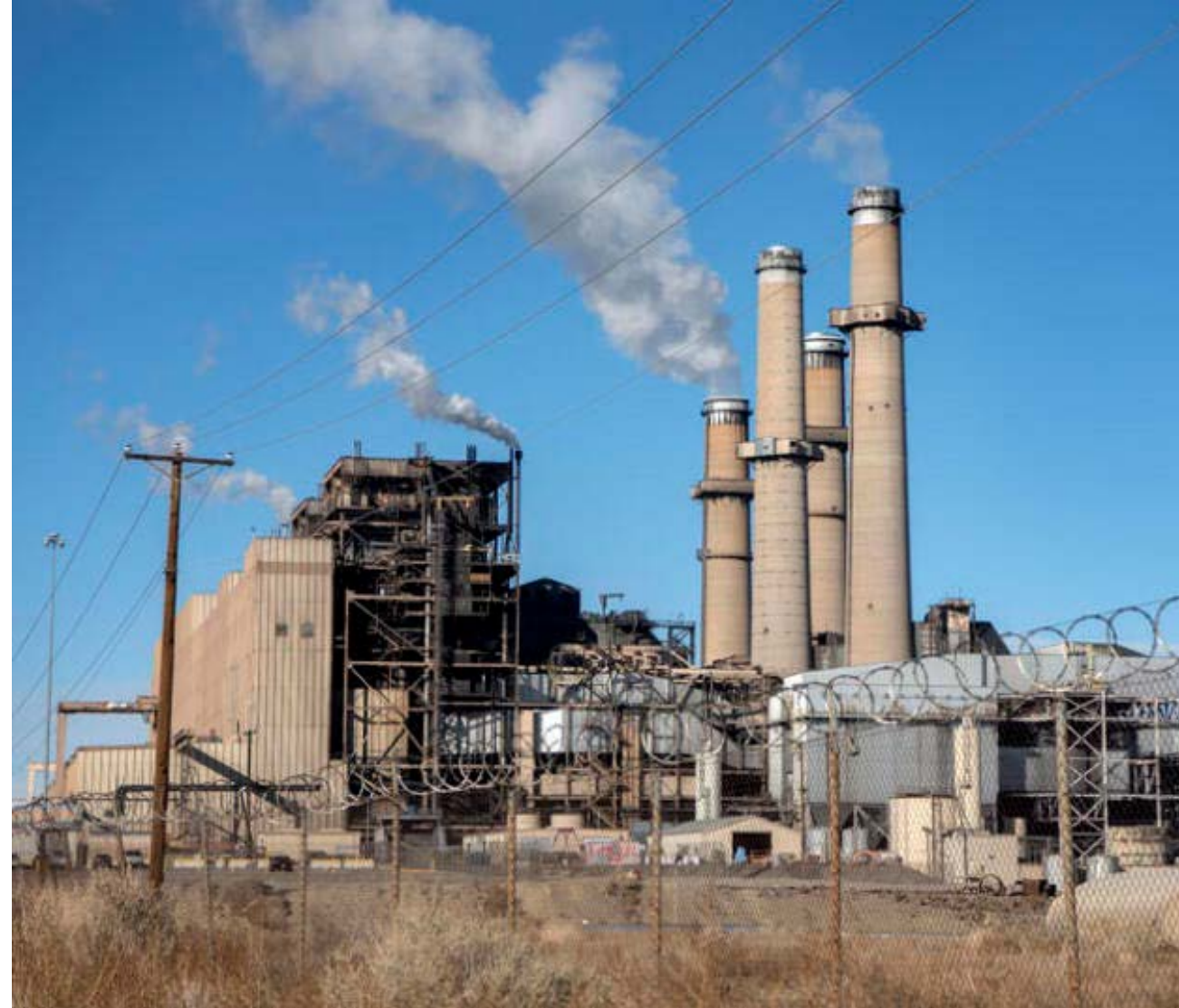
San Juan Generating Station Photo Credit: The Albuquerque Journal
