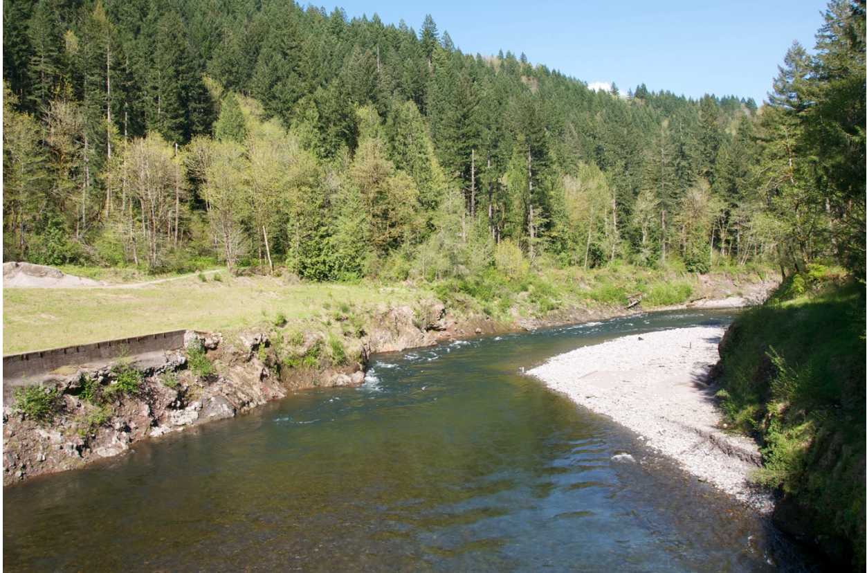
Former Marmot Dam Site, Sandy River, Oregon
